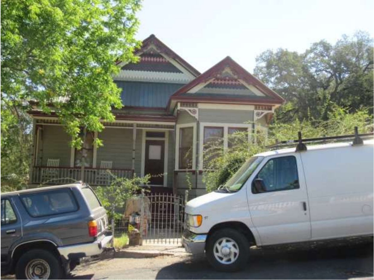
Church Street (work in progress).
