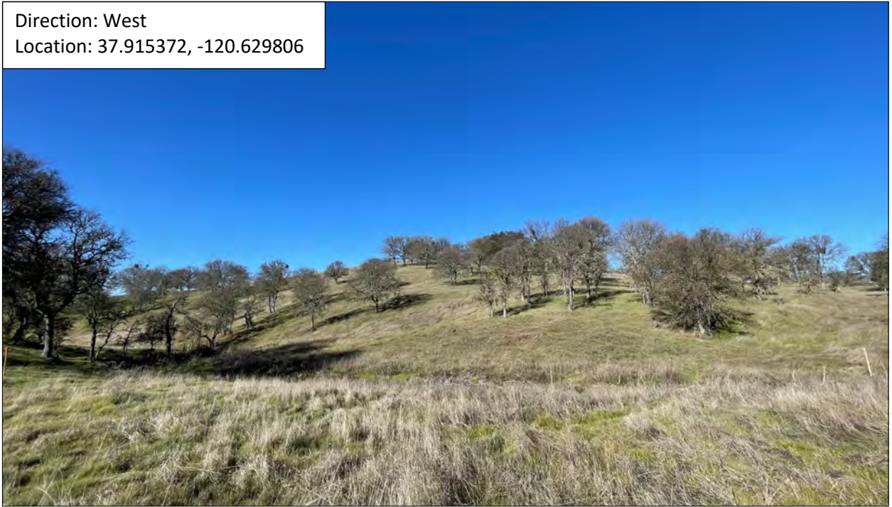
Photo 1. Looking west from Photo Point 1 at the proposed access road stream crossing.
