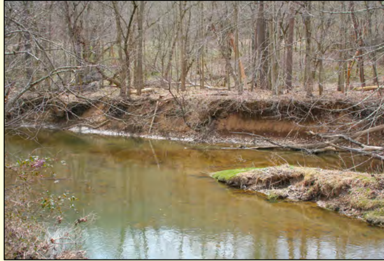
Exhibit 3-10: Stream bank erosion from stormwater. Heavy flows have scoured the bank of Whiteley Creek in Garards Fort, Pennsylvania, leaving roots exposed, toppling trees, and increasing the amount of sun falling on the stream, which raises the water temperature. Photo source: EPA
