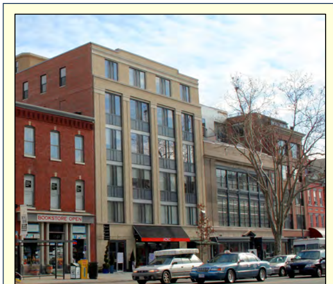
Exhibit 4-2: Infill development. Developers of the Matrix Condos in Washington, D.C., converted a long-abandoned former auto dealership into a mixed-use project by building on adjacent empty lots and adding two stories to the existing building, set back from its façade. The condo residents are within walking distance of downtown, a grocery store, multiple restaurants, and other local businesses. A bus stop is right outside their front door.
